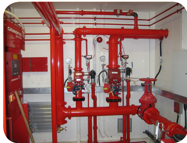
FIRE WATER LINE WORKS
