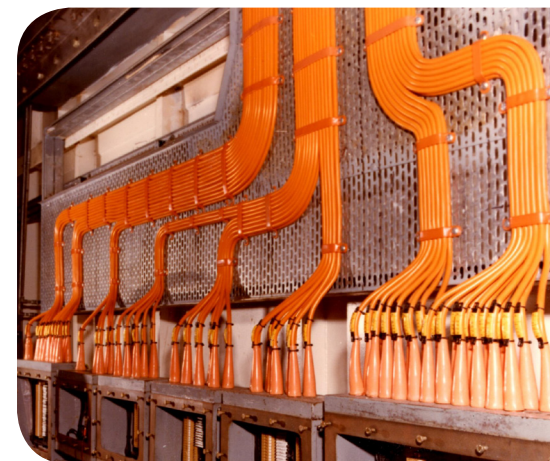
MICC CABLING WORKS
