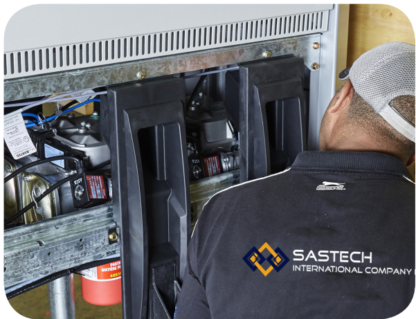
FUEL STATION MAINTENANCE WORKS
