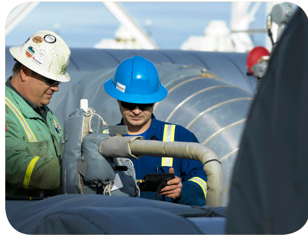
GAS LINE WORK & MAINTENANCE
