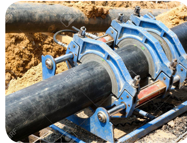
HDPE PIPING WORKS
