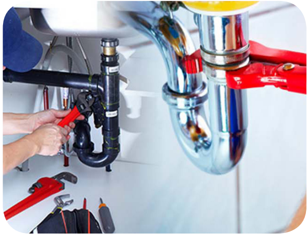
MEP WORKS & MAINTENANCE
